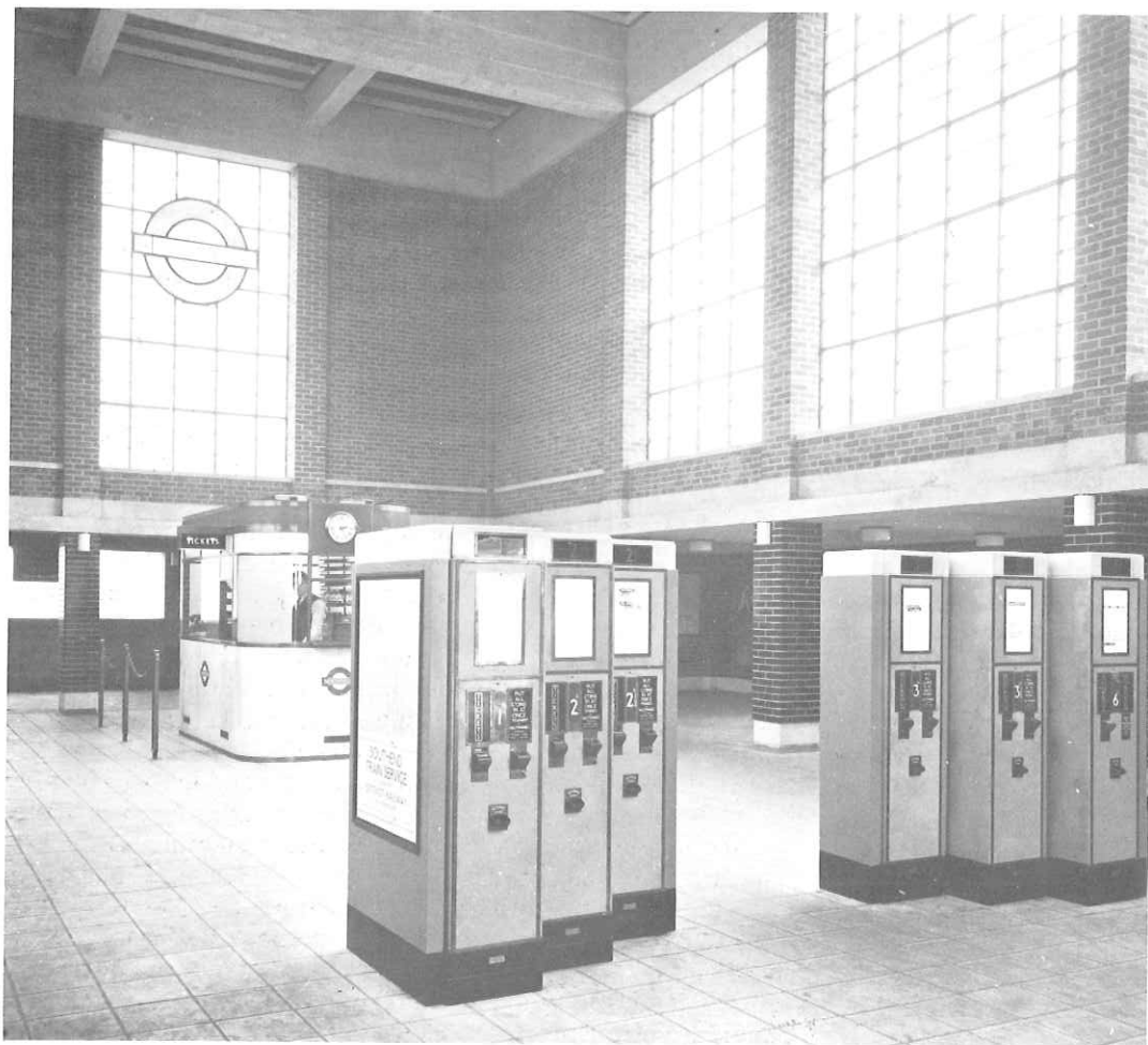
Ticket Hall, Northfields station, 1933. The clerestory lighting system extensively used by the architect, Charles Holden, for the new Underground stations served to light the stations internally by day, and advertise them externally by night.
