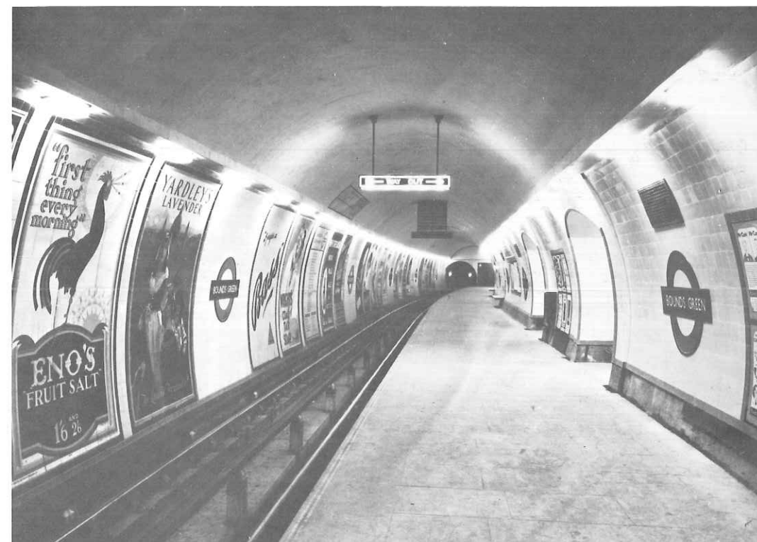
Platform, Bounds Green station, in 1932. The improvements to station design gave the platform tunnel a smooth shell, improved the lighting, and clearly distinguished station signs from posters.
